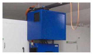
Refrigerating machine in the installation room (possibly cooling of the emitted heat is required)
