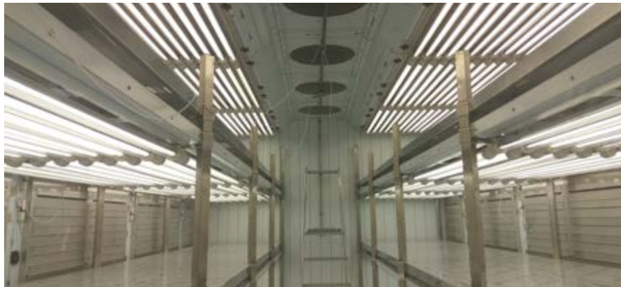
Plant Growth Cabinet with Lamp Shelves (approx. 16 KW waste heat of lighting)
